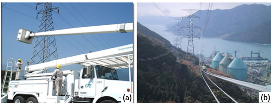
Fig. 1 a Workers checking with climbing equipment [10] b Workers performing preventive maintenance on transmission lines suspended tens of meters above the ground [11]
