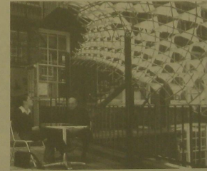
Picture 3. Limited Membrane Structure shaped according to Sun light, Wind and Rain Analysis
