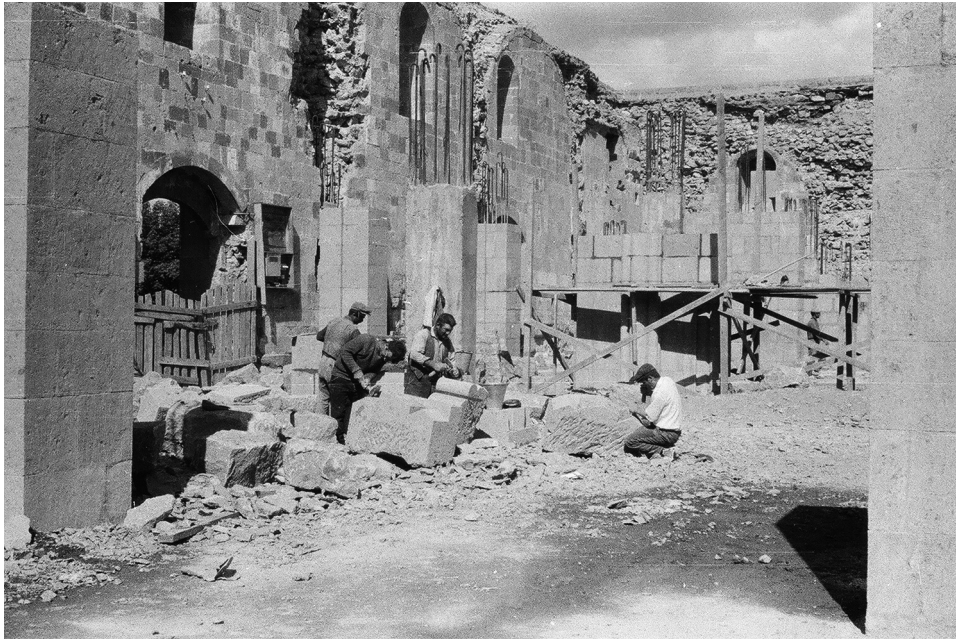
Figure 15. Restoration of the grand mosque of Erzurum in the 1960s with stone masonry and RC techniques side by side (source: VGM archive, https://www.vgm.gov.tr/kurumsal/vakif-kayitlar-arsivi/vakif-kayitlar-arsivi ).
