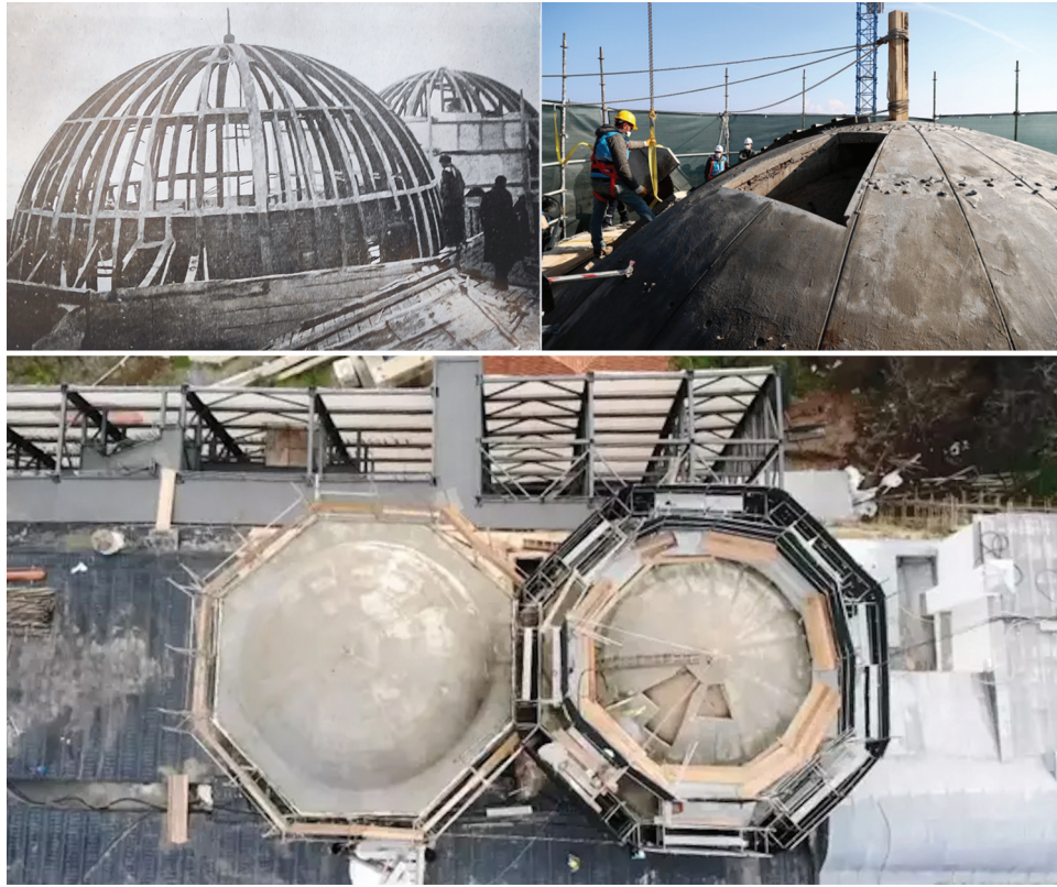
Figure 14. Topkapı palace, Fatih Mansion: conversion of original timber dome to RC dome in 1942 and its dismantling in 2021 (sources: Öz 1991, 51 [top left]; Ergör and Benlioğlu 2021 [top right and bottom]).
