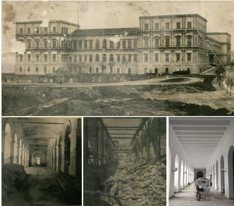
Figure 10. Substitution of wooden elements with reinforced concrete at Taşkışla, an Ottoman military building converted to the faculty of architecture of Istanbul Technical University in 1944 (source: encümen archive file No. 1107, Istanbul regional board of conservation of cultural heritage [Istanbul technical university faculty of architecture Taşkışla building]).
