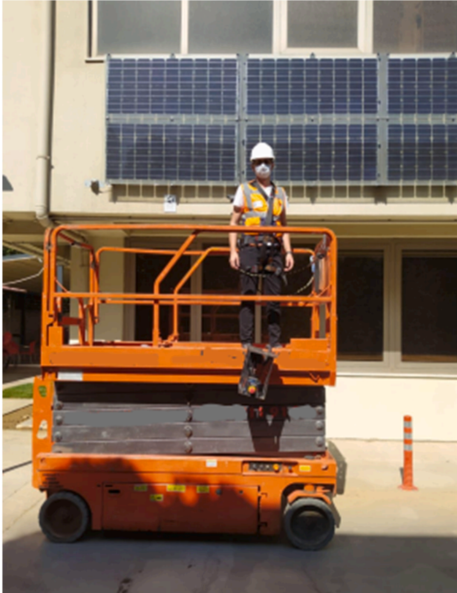
Fig. 5. Example from field observation of working at height.
