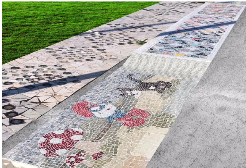
Figure 10: Mosaic bank, prepared by Demirkol, the project manager and consultant, with waste porcelains
